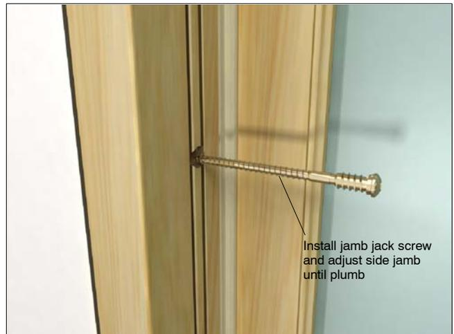
**Figure 7: Install jamb jack and plumb jambs**
