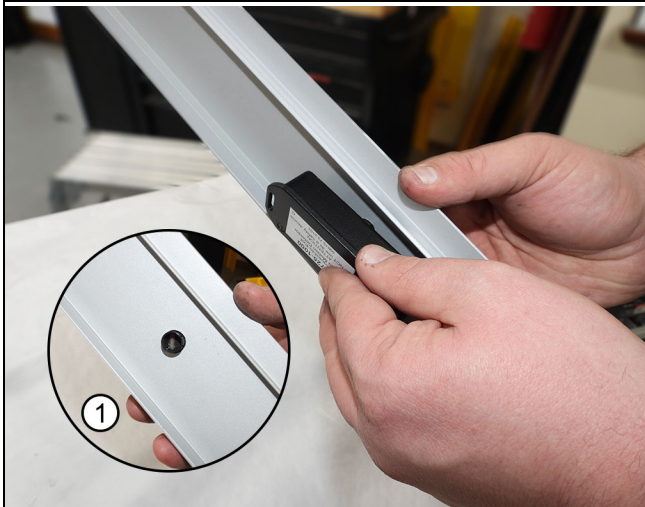
Figure 34 Inset shows sensor eye through head jamb cover
