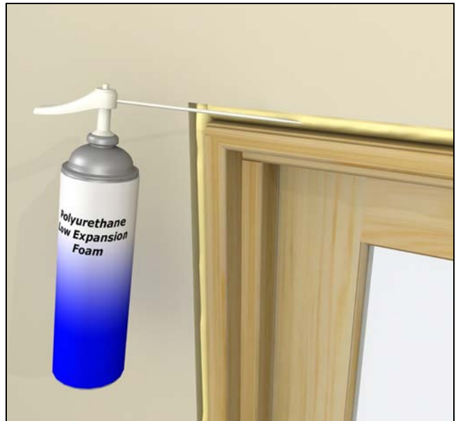
Figure 20 Apply low expansion foam between frame and rough opening.
