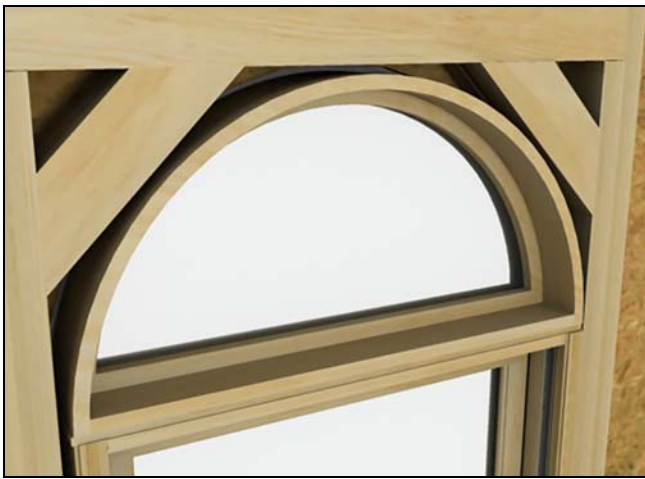
Figure 3 Typical rough opening for a round top.
