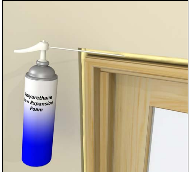
Figure 21 Apply low expansion foam between frame and rough opening.
