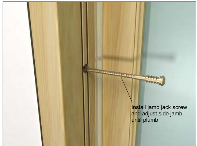
Figure 7: Install jamb jack and plumb jambs
