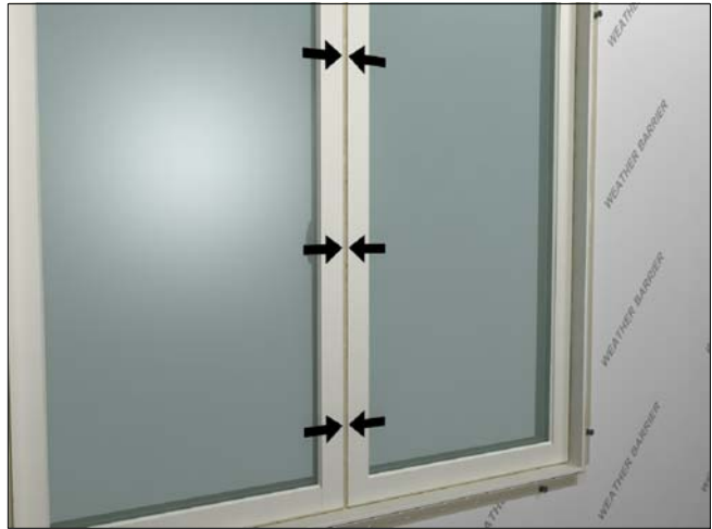
Figure 10: Adjusting the reveal between the sash
