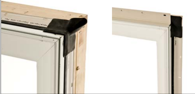
Figure 3 Preparing the unit for installation.
