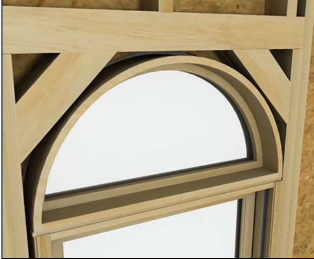
Figure 2 Typical rough opening.
