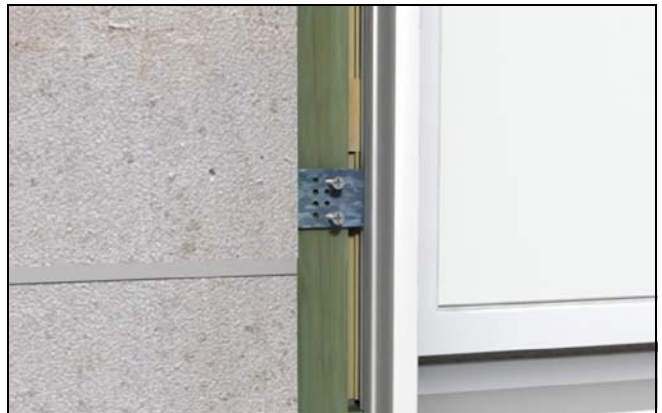
Figure 19 Attaching window with structural brackets.
