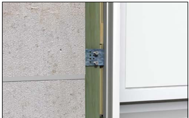
Figure 19 Attaching window with structural brackets.
