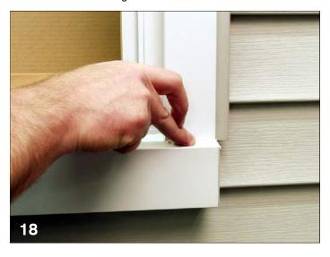
27. Seal the joint between panning components and exterior of building with compatible sealant. See figure 19. Be sure to tool out bead for best performance.
