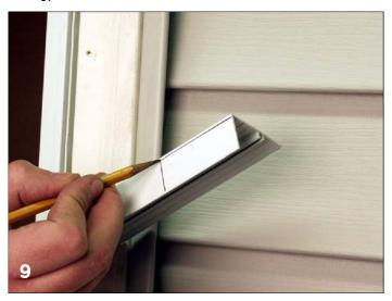
15. With a hacksaw, cut a notch on lines and remove any burrs with a metal file. Test fit the piece to make sure it fits around jamb casing. Some trimming may be necessary.
