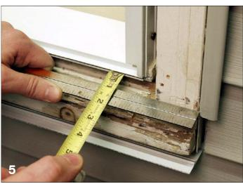
8. Extend these marks at right angles until they intersect. Cut an additional 1/16" notch from the back side of the sill panning notch. This will allow clearance for the jamb panning once installed. With a hacksaw, cut a notch in the sill panning and remove any burrs with a metal file. See figure 6. Test fit sill panning to make sure it fits properly around existing jamb casing. Some trimming may be necessary.
