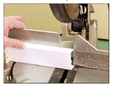
Measure from top of sill to bottom of head jamb panning. Cut jamb panning components to this measurement with a power miter saw or hacksaw. See figure 12.
