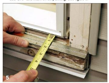
8. Extend these marks at right angles until they intersect. With a hacksaw, cut a notch in the sill panning and remove any burrs with a metal file. Remove an additional 1/16" from the back side of the sill panning. This will allow clearance for the jamb panning. See figure 6. Test fit sill panning to make sure it fits properly around existing jamb casing. Some trimming may be necessary.
