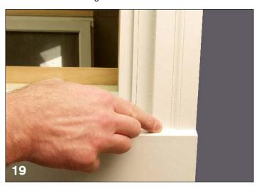
26. Seal the joint between panning and exterior of dwelling with compatible sealant. Be sure to tool out bead of sealant for best performance.
