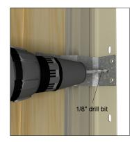
1. Install clips at the recommended locations as shown at the beginning of this instruction. Place the short end of the bracket on the back side of the nailing fin. Attach the clips to the wood jamb liner with the three #7x 5/8" screws provided.
