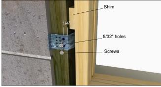
Figure 9 Attaching window with masonry clips or structural brackets.
