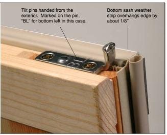
Figure 2: Replacing tilt pins and bottom sash weather strip
