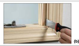
Figure 15: Removing Ultimate Casement stops and covers.
