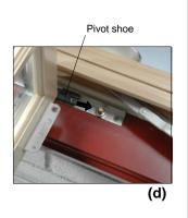
Figure 18: Removing Ultimate Casement Operator Sash
