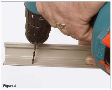
NOTE: The first screw on both the top and the bottom will need to be located 2" from each end.
