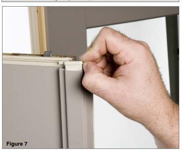
NOTE: Until the bottom end cap is in its position, the astragal weather strip will have a tendency to slide downwards.
